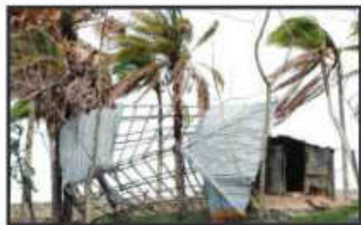
The wind is blowing the roof away.
