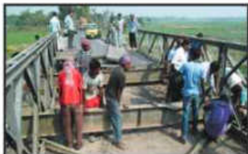
The workers are repairing the bridge.
